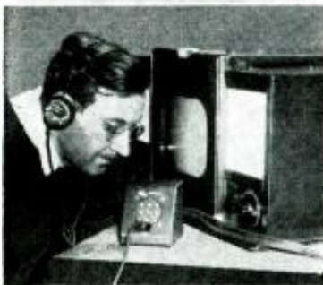
When more than one man is on the installation the extra set of headphones plugs into the "downstairs" cabinet for two-way communications without the necessity of a separate transmission line.
