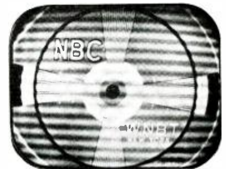
Fig. 2—Bars caused by interfering ham or FM.
